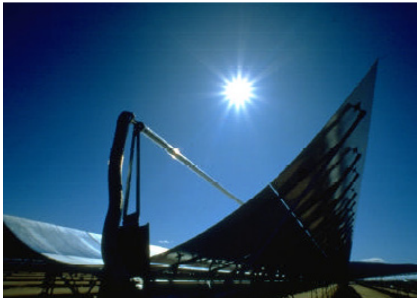
Figure 41 : Parabolic reflectors producing electricity used for hydrogen production
